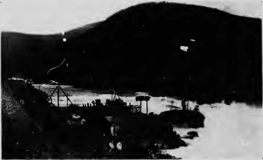
Kootenay River Development. Bonnington Falls Plant No. 1 at Lower Bonnington Falls.
